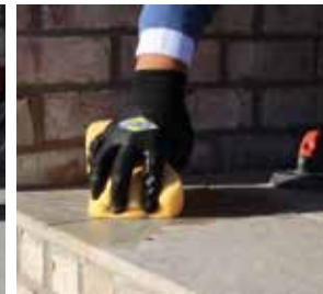
PIC 2. Remove excess grout with clean water.
