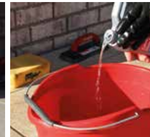
PIC 3. Add specific acid cleaning agent for porcelain tile to clean water.
