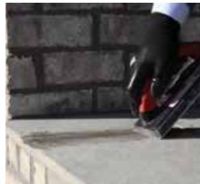
PIC 1. Fill joint with grout.
